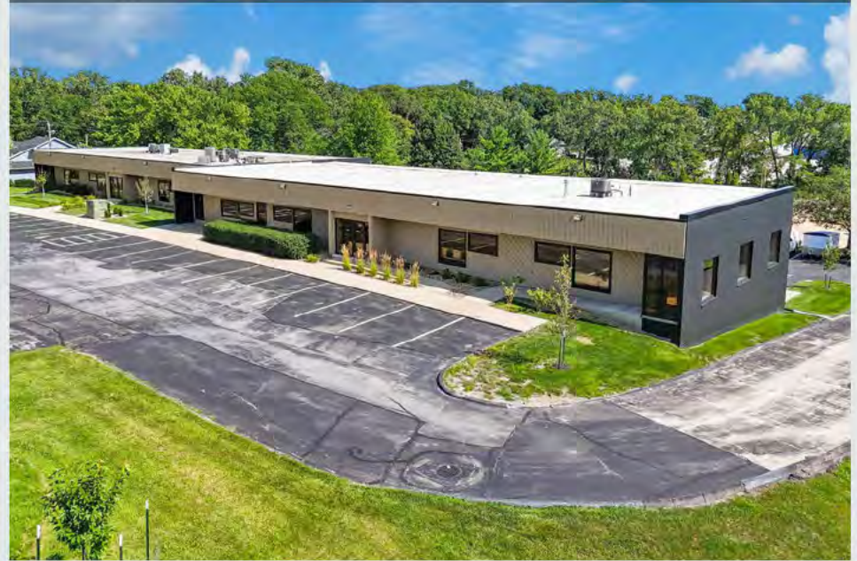
Upper Level - North Side
